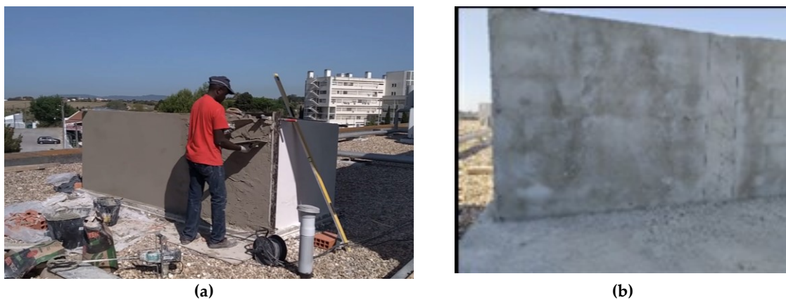
Figure 4.4 Mortar at the South-facing wall: (a) application of the outer layer; (b) Inner layer.
