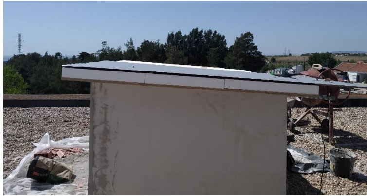
Figure 4.6 Construction of the roof of the test cell.
