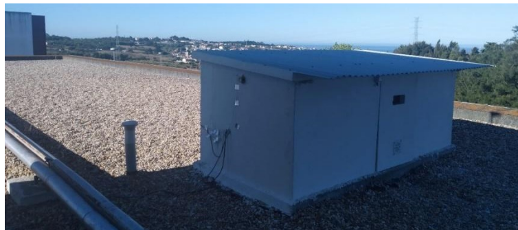
Figure 4.7 North-facing wall of the test cell.
