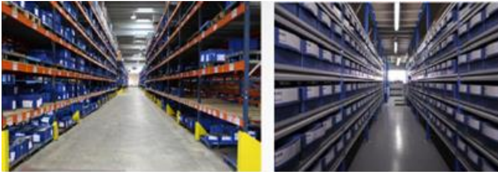
Appendix 16 Examples of Industrial Racking
