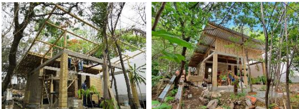
Figure 5. Example of educational and training activities and application to modern building with Compressed Earth Blocks. Source: Bienal de Arquitectura de Chiapas.
