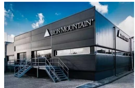
IRM Data Center facility.
