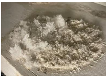
Figure 26 Plaster board after use, left for a few days, salts starting to accumulate. (©Nour Ali)
