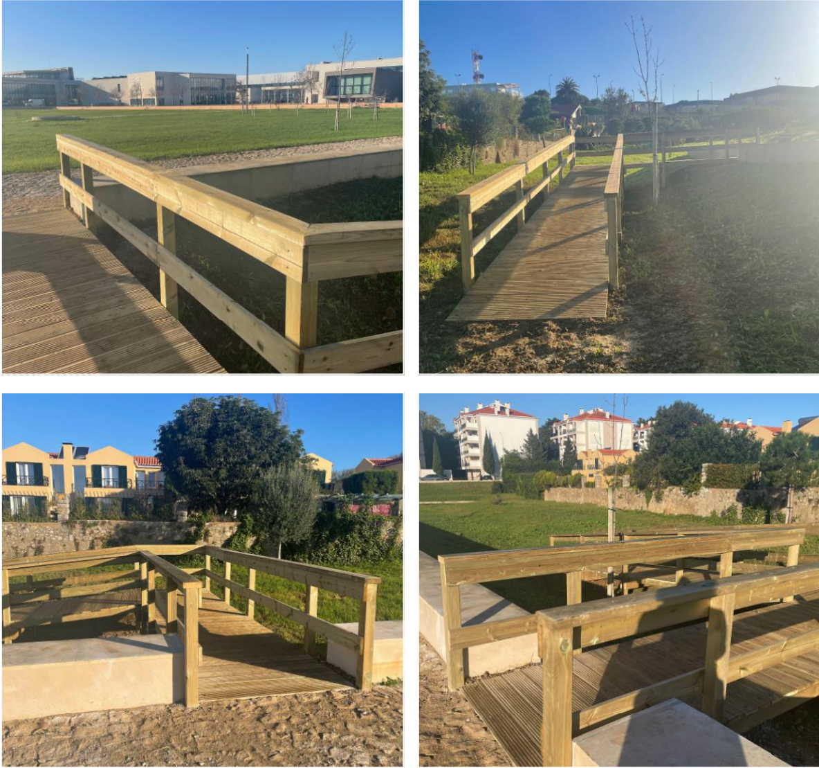
Figure 13: Physical Space – Cascais built a ramp for an inclusive access of the community garden at Nova SBE
