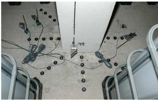
(a) Strengthened interior connection C2-1
