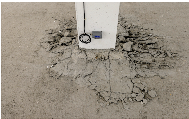
(a) As-built interior slab-column connection B2-1
