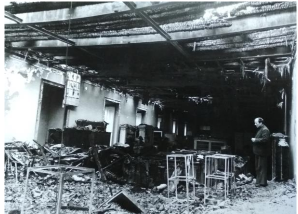
Figure 1.4 – Former geology room after the fire of 1978. Photographs by Professor Fernando Barriga.
