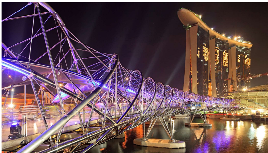
Figura 1.1: Helix Bridge, Singapura (fonte: www.arup.com/projects/helix-bridge ).
