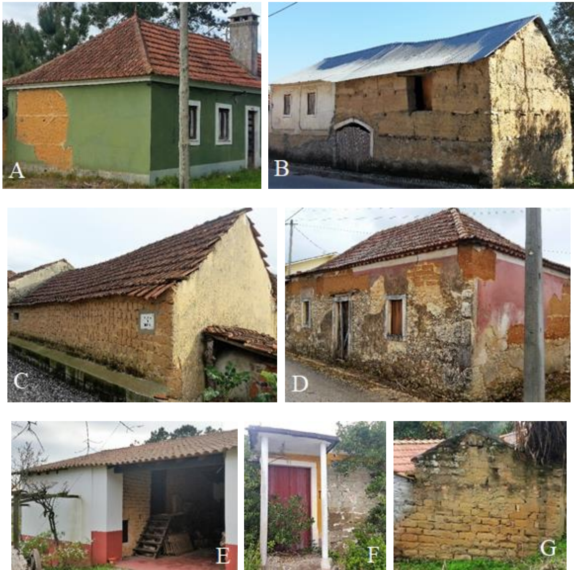
Figure 3. Some of the 98 mapped and inspected vernacular earthen buildings: A – rammed earth building 77 from Pombal; B – rammed earth building 10 from Pombal; C – adobe building 65 from Leiria; D – mixed construction 38 from Pombal; E – adobe building 93 from Leiria; F – adobe building 87 from Leiria and G – adobe building 42 from Leiria
