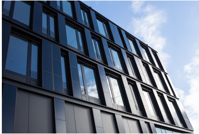
Figure 0.2: A PV facade of a building constructed by ZSW in Stuttgart[23].
