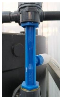
Figure 8: Venturi tube photo
